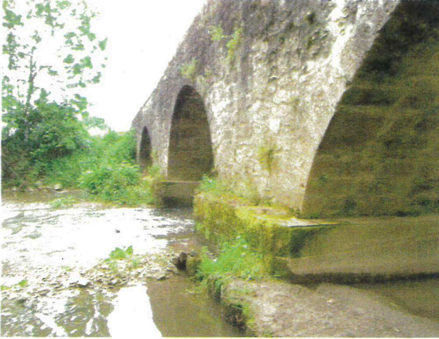
Face amont. Photo UDAP46.
