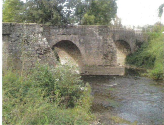
Face aval. Photo UDAP46.
